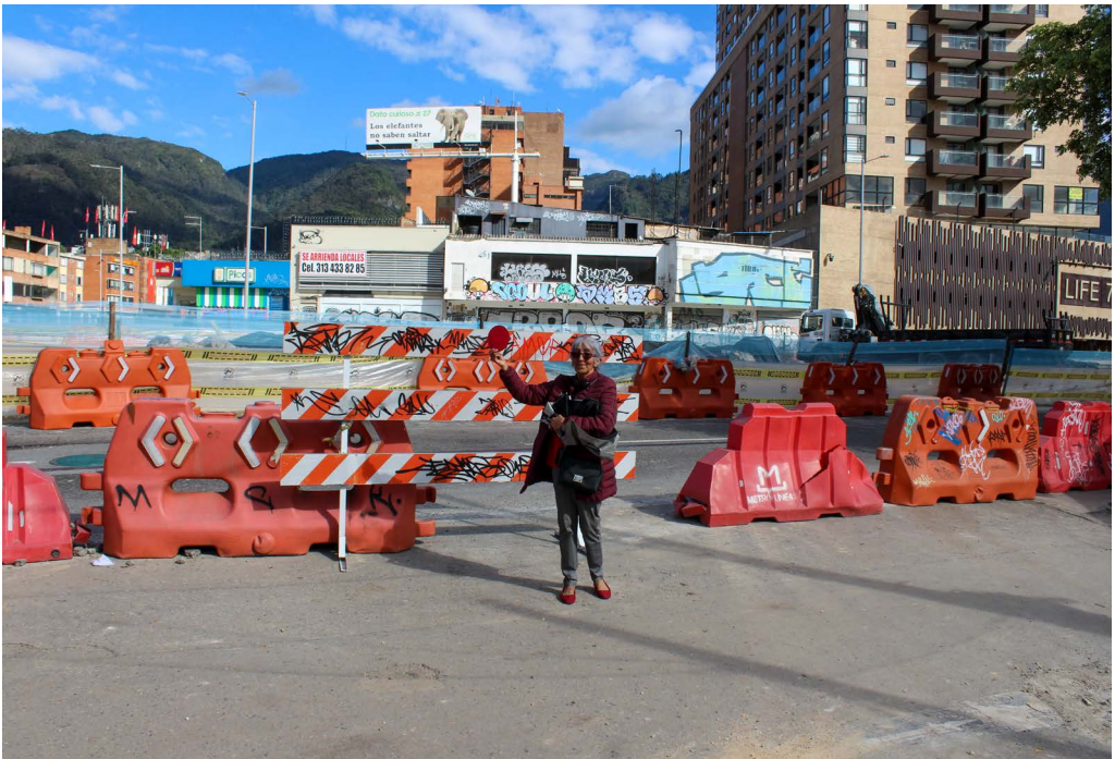
Construction site in Barrio Nuevo, showing the inaccessibility of the public realm.
