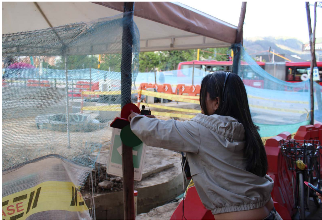
Participants “tagging” unsafe construction site conditions.
